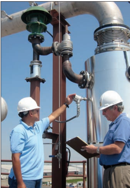
Patrick Samson, assistant plant manager (left), discusses the plant's operation while out in the main yard with Plant Manager Bruce Cohen.
